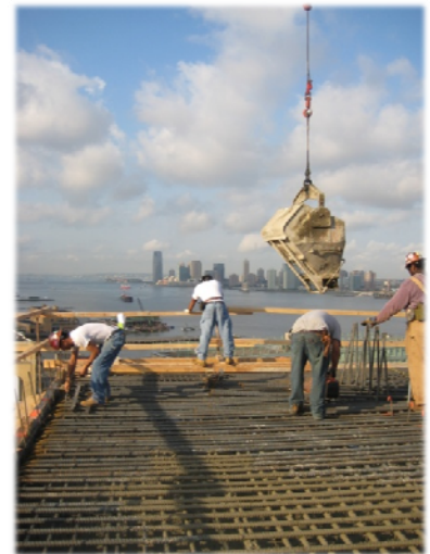
Figure 19: Heavily-reinforced 19th floor transfer slab
