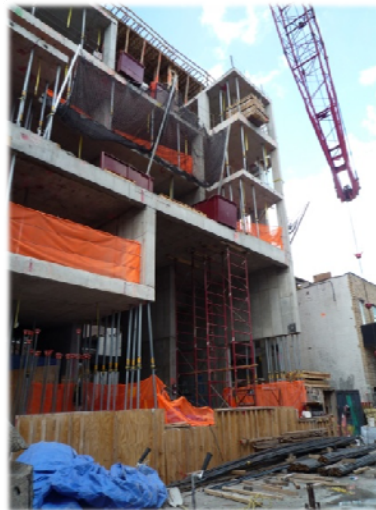
Figure 18: Cantilevered slab as part of balcony system
