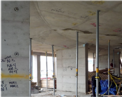
Figure 17: View of transition from 9" slab to 18.5" slab
