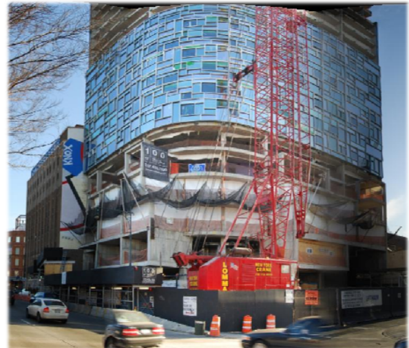
Figure 57: View of panelized facade from south-west corner
